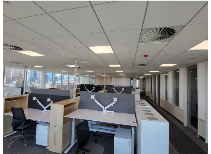
Furniture installation in office levels
