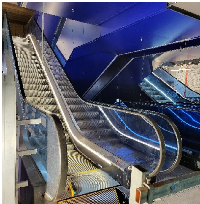
Internal escalators installed
