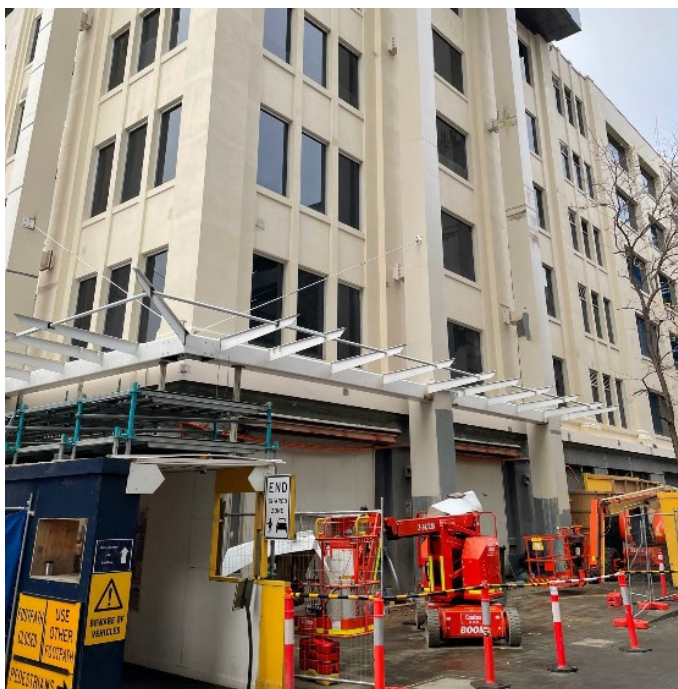
Young St Glass Canopy in progress
